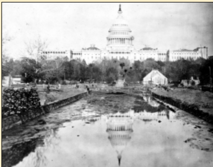
A view of the Washington Canal in the 1860s, fouled with silt, debris, refuse, and sewage.
