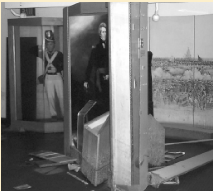
Storm damaged displays at the Jean Lafitte National Historic Park.
