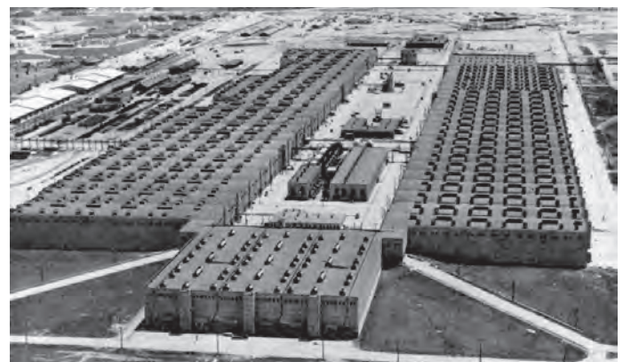
K-25 aerial view
