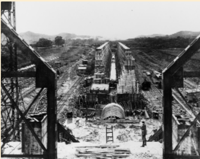
The Pedro Miguel locks under construction at the Panama Canal, January 1911.
