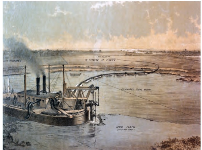
Cutterhead dredge at work in Oakland Harbor, 1884
